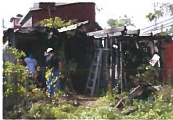
August 2012 north shed removal by Troop 25.
